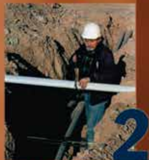
Step 2: Cut Split Duct Conduit to Fit
