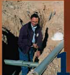
Step 1: Remove Damaged Conduit
