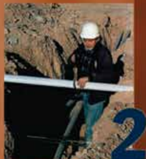
Step 2: Cut Split Duct Conduit to Fit
