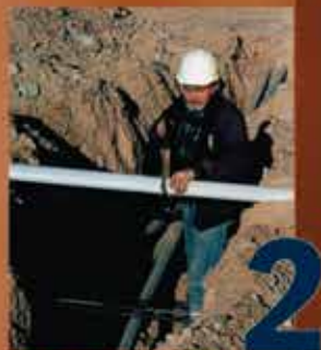
Step 2: Cut Split Duct Conduit to Fit
