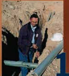
Step 1: Remove Damaged Conduit
