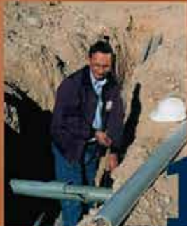
1 Step 1: Remove Damaged Conduit
