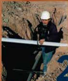
2 Step 2: Cut Split Duct Conduit to Fit
