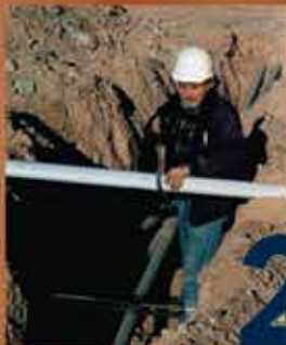
2 Step 2: Cut Split Duct Conduit to Fit
